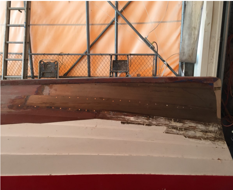
NEW PLANKING INPLACE ON THE STERN OF THE ERICA
